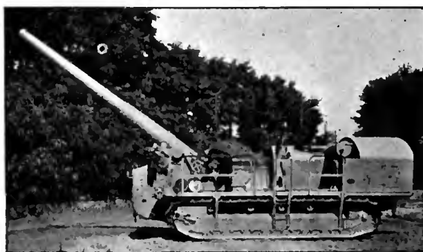
FIG. 32.—French 220-mm. Schneider, caterpillar carriage.
