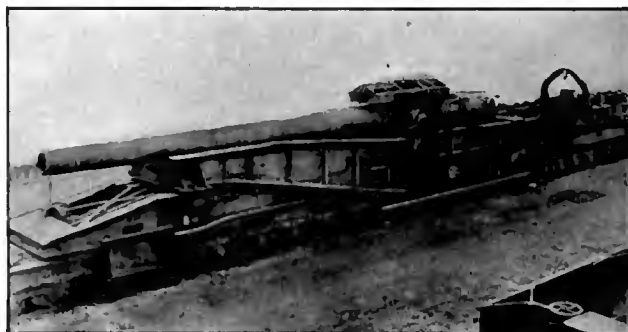
FIG. 45.—German 380-mm. gun, on railway mounting.
